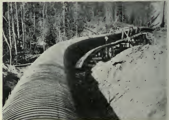
Fig. 5—66" Wood Stave Pipe Syphon, Kamloops Power Plant.
